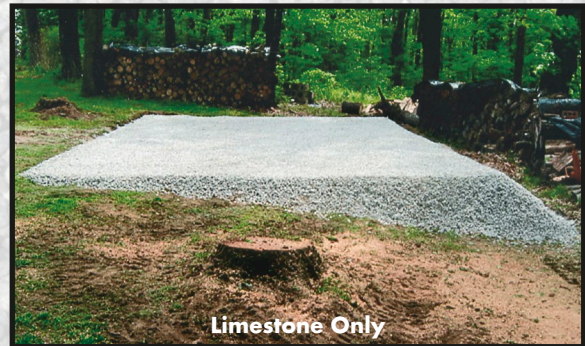
Sod dug out 4" with limestone on top to ground level Does not include hauling out sod. Hauling out sod is available for an additional fee.
