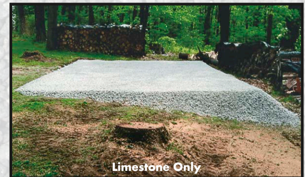
Sod dug out 4" with limestone on top to ground level Does not include hauling out sod. Hauling out sod is available for an additional fee.
